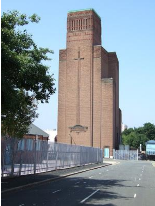
One of Rowe's ventilation towers (Birkenhead)
