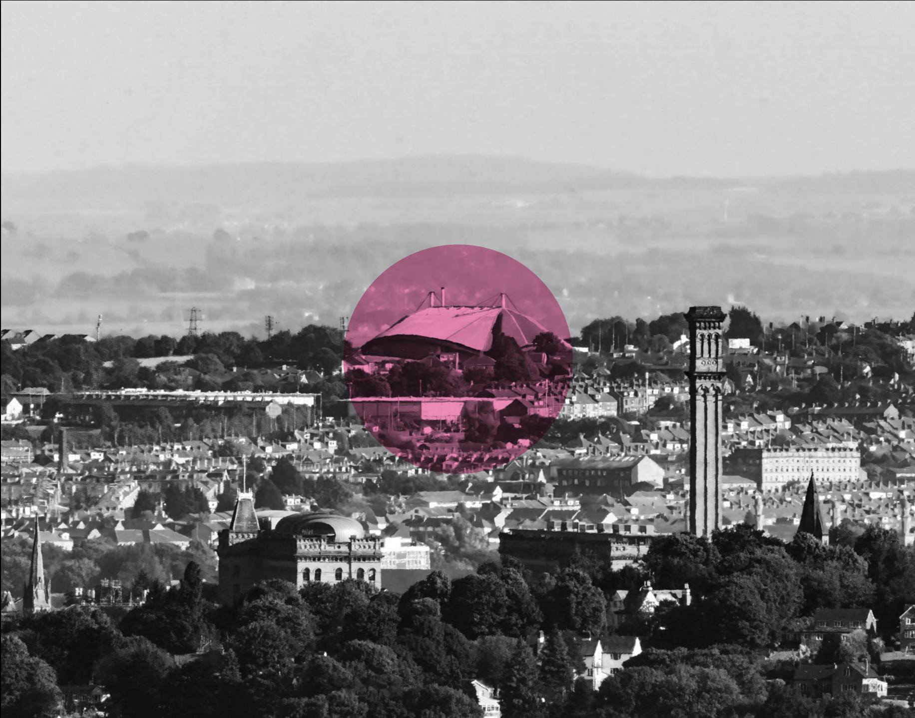
The 'big top' of Richard Dunn Sports Centre on the Bradford skyline, with the chimney of the 1873 Lister Mills in the foreground.
