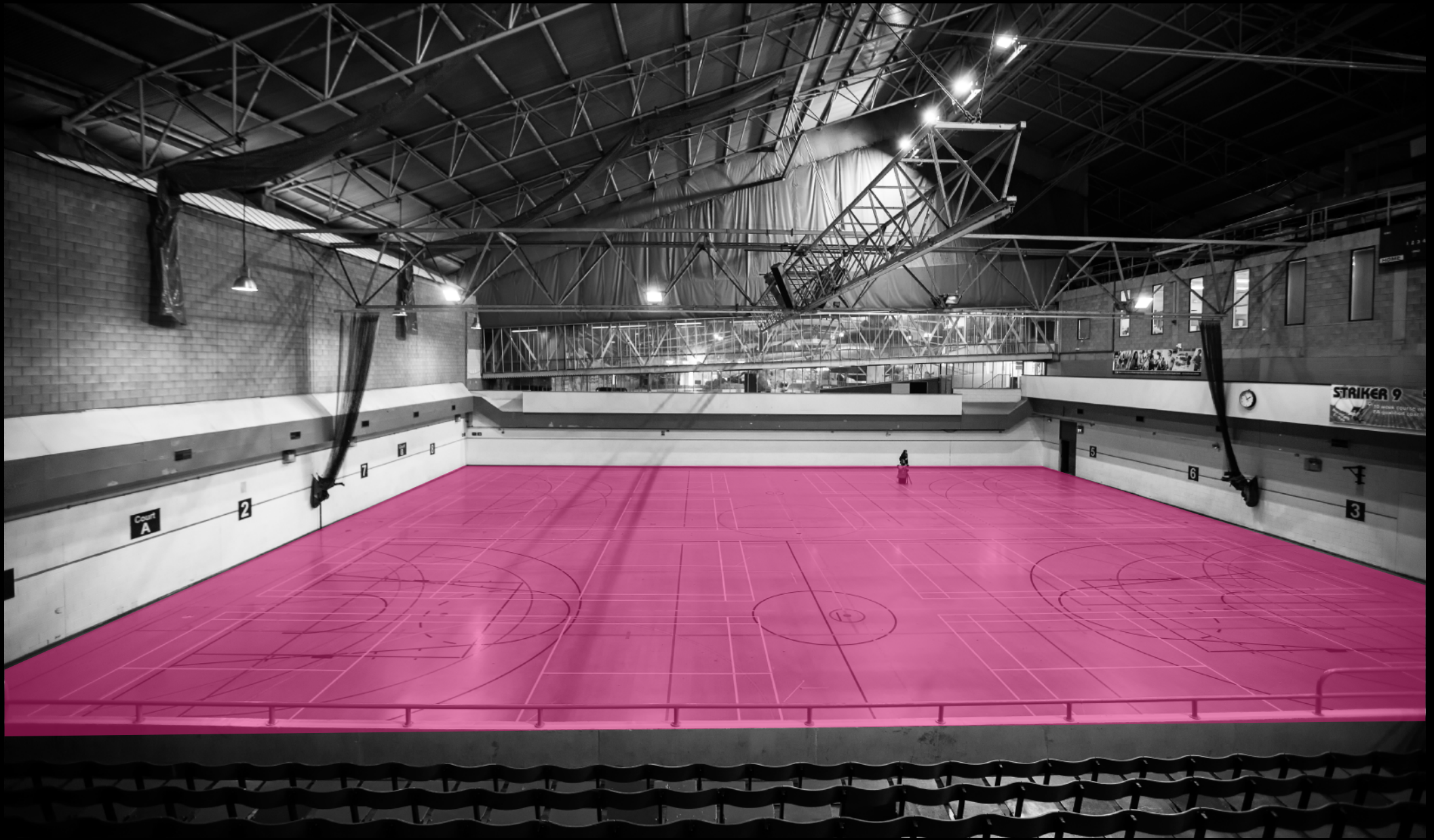
The former sports hall would become a 1475m 2 indoor/outdoor arena for skateboarding and wheel sports, with timber ramps, rails and obstacles.
