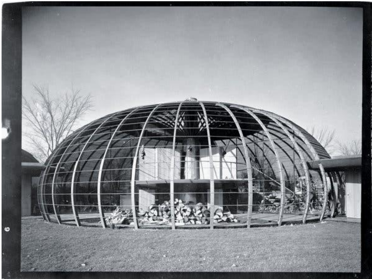
The back of the Ford House in Aurora, Ill., reveals Quonset hut ribs. Credit... Bruce Goff Archive, Ryerson and Burnham Archives, the Art Institute of Chicago
